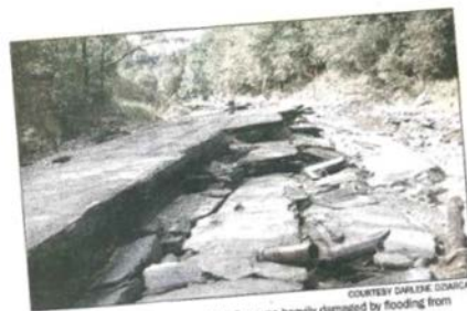
ROUTE 2 between Cropseyville and Grafton was heavily damaged by flooding from Tropical Storm Irene. Officials said portions of the road were badly damaged.
